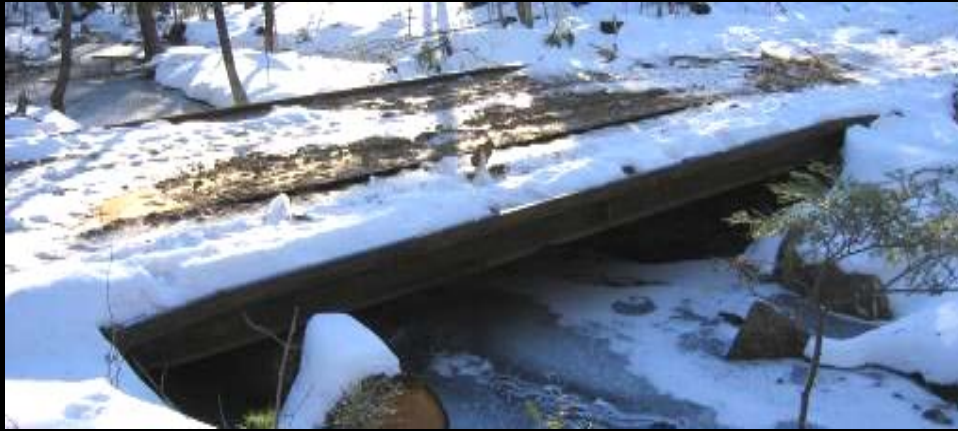
Temporary Bridge Deck
