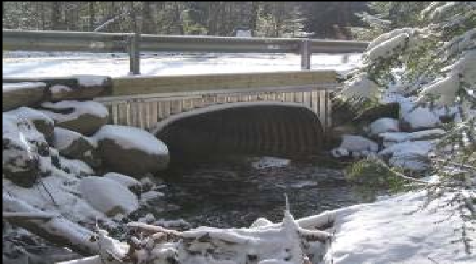
Bottomless Box Culvert
