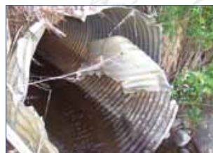
damaged culvert
