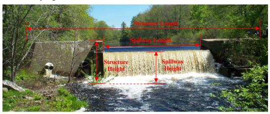
Taking measurements of dams can be difficult even in periods of low flow, so proceed carefully, and make estimates when necessary. If measurements cannot be taken directly, please estimate and write EST after any estimated measurement. If <u>all</u> dimensions are either measured or estimated, check the box provided. You can use the *Site Sketch* area on the back of the field form to record additional dimensions or dam features.
