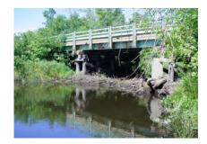
Debris Jam may be composed of a mixture of large and small trees, logs and much smaller woody debris that has naturally accumulated with few if any signs of beaver cut pieces. Such jams will often extend only part of the way across the channel, and may be passable
