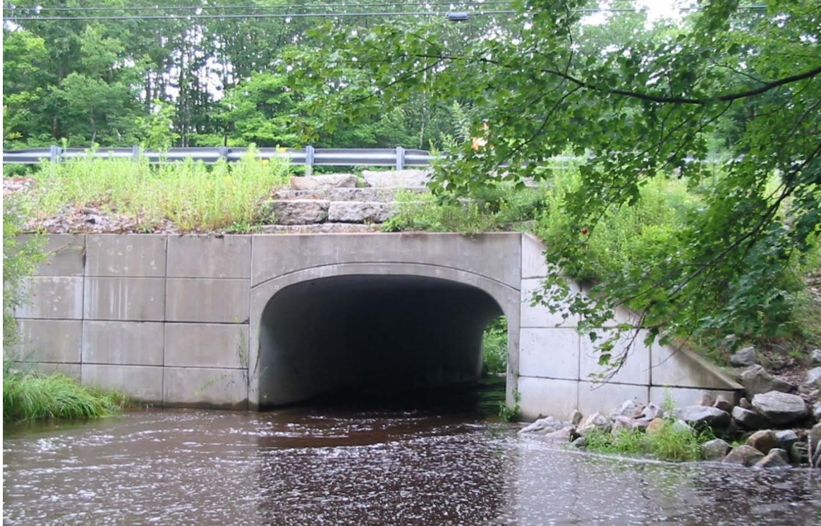
Bridge over Ward Brook on Alewife Road in Kennebunk.
