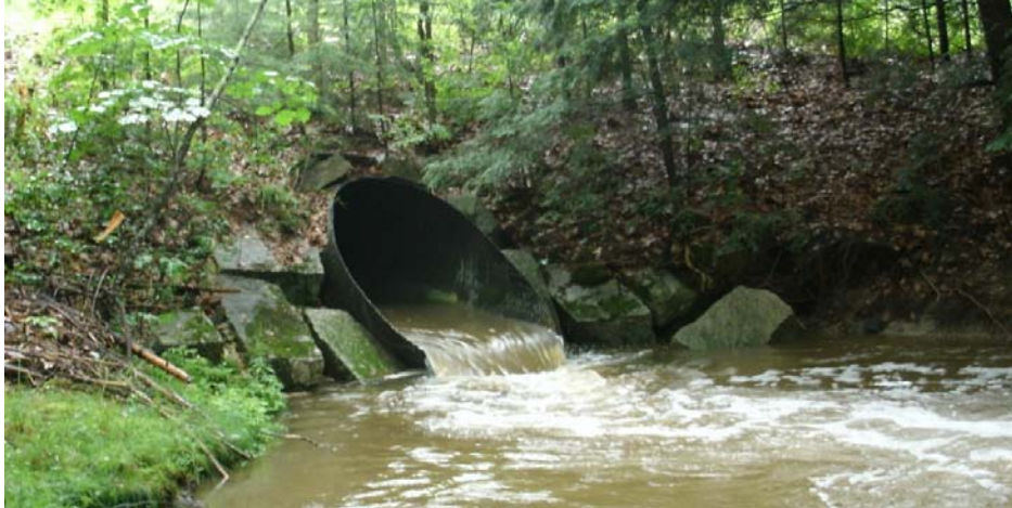
Perched Outlet at Duck Brook crossing on Limerick Road in Arundel.
